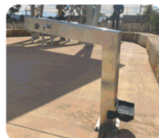
ACCESSIBLE DRINKING FOUNTAIN With bottle refill and dog bowl - located 10m min. from playspace.
