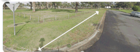
1.5m wide concrete footpath connecting to existing pram ramp on Collins Street
